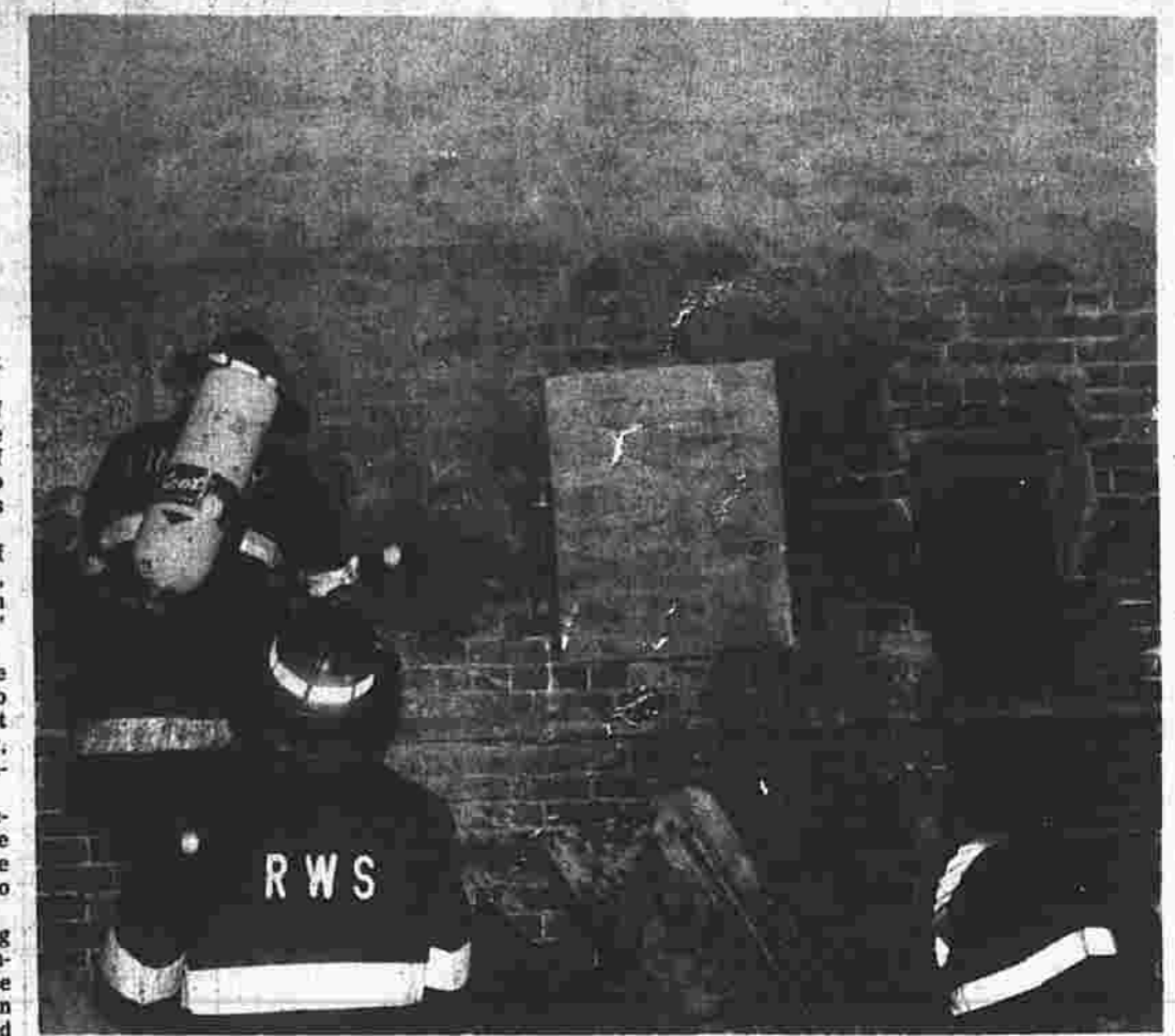
Firefighters from the Town Fire Department used only minor damage to the tunnels and none to the building above.
